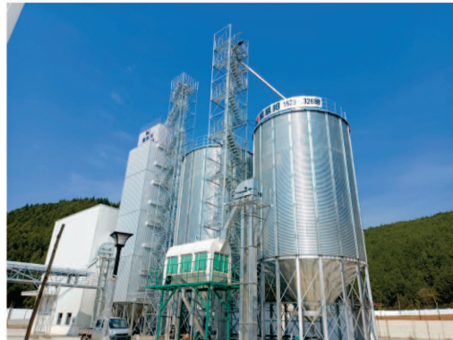
全钢锥底筒仓 All steel cone bottom silo
